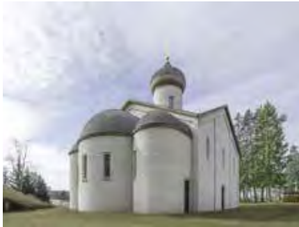
Tchoban Voss Architekten, Sergei Tchoban, Germany, Russian Monastery Of St George Goetschendorf, Milnersdorf-Goetschendorf, Germany, 2017
