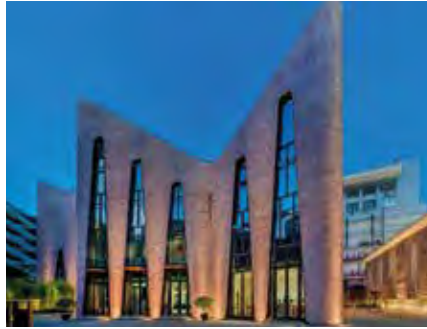
INUCE, Dirk U. Moench, Switzerland, Urban church of Huaxiang, Fuzhou City, Gulou District - Fujian Province, China, 2018
